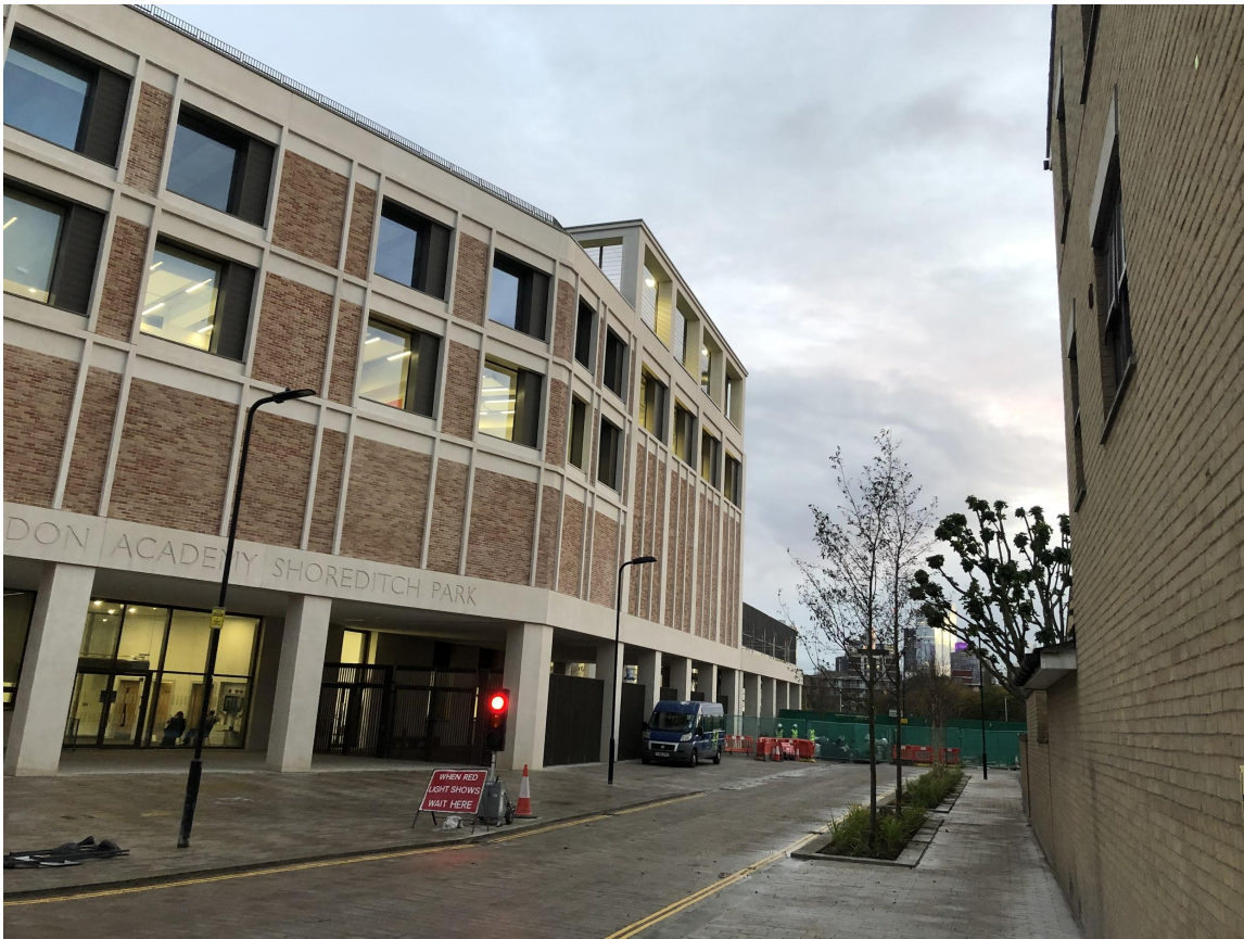
View south alongside Phase 1 school building (left):
